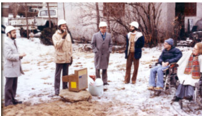
3710 Chicago Groundbreaking January 16, 1980
