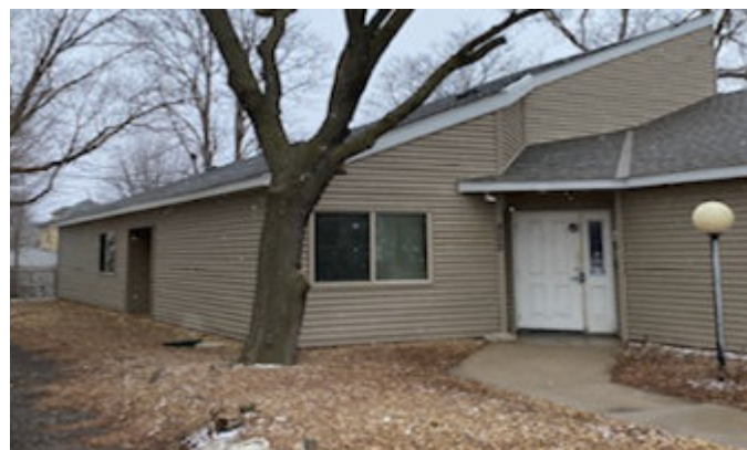
New siding at the Iglehart House
