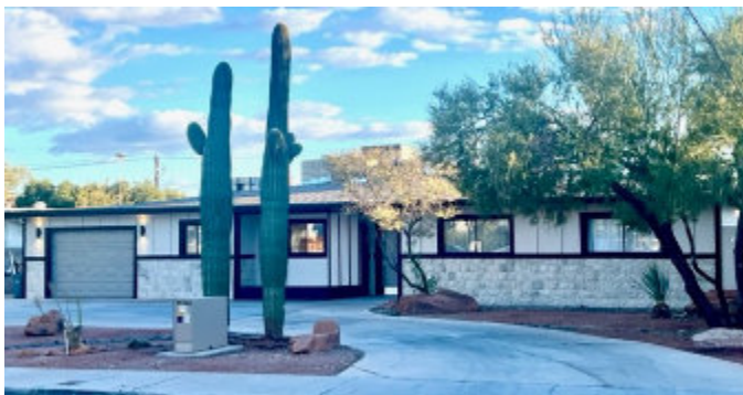
Updated front façade of Hastings House
