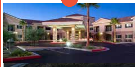
Coronado Drive Apartments opened, a 60-unit building for seniors in Henderson, Nevada.
