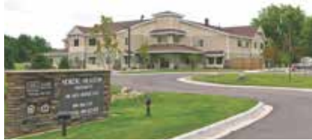
ASI's 39th building in Minnesota opened: Nordic Meadow Apartments in Alexandria.
