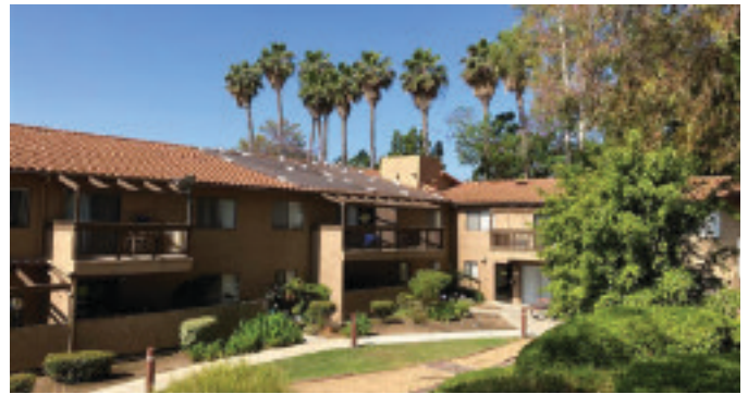
New roof being installed at Harbor View Terrace in Fullerton, California.
